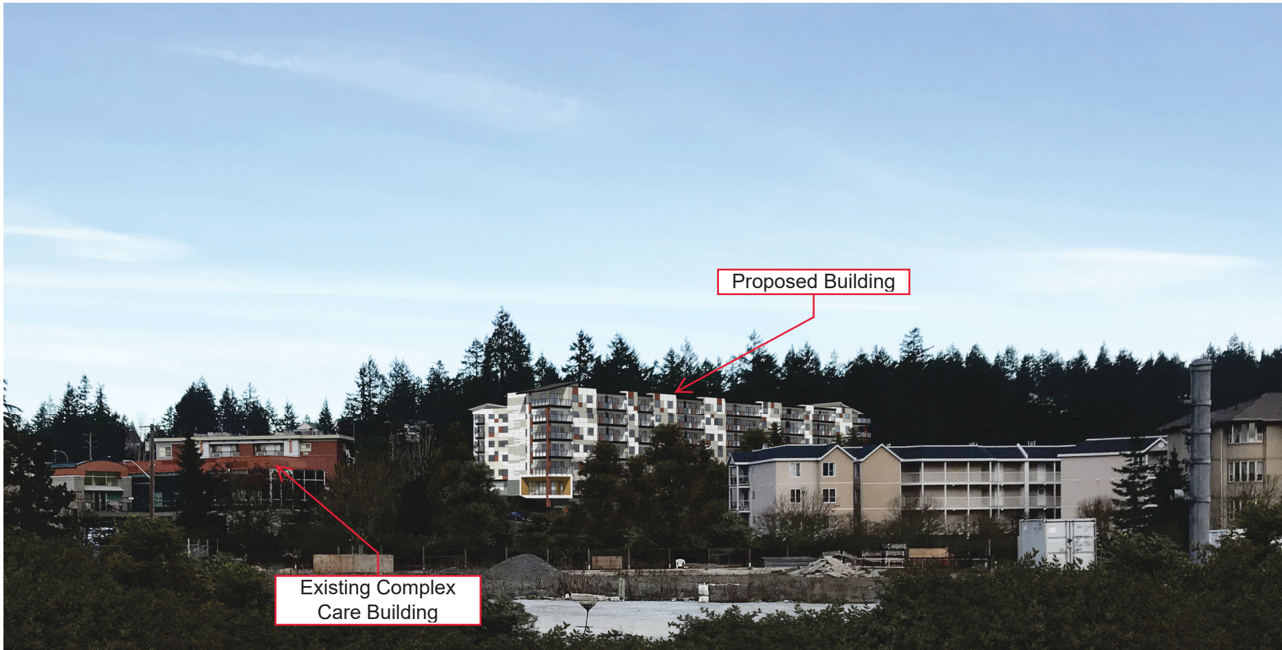
VIEW FROM ISLAND HIGHWAY
